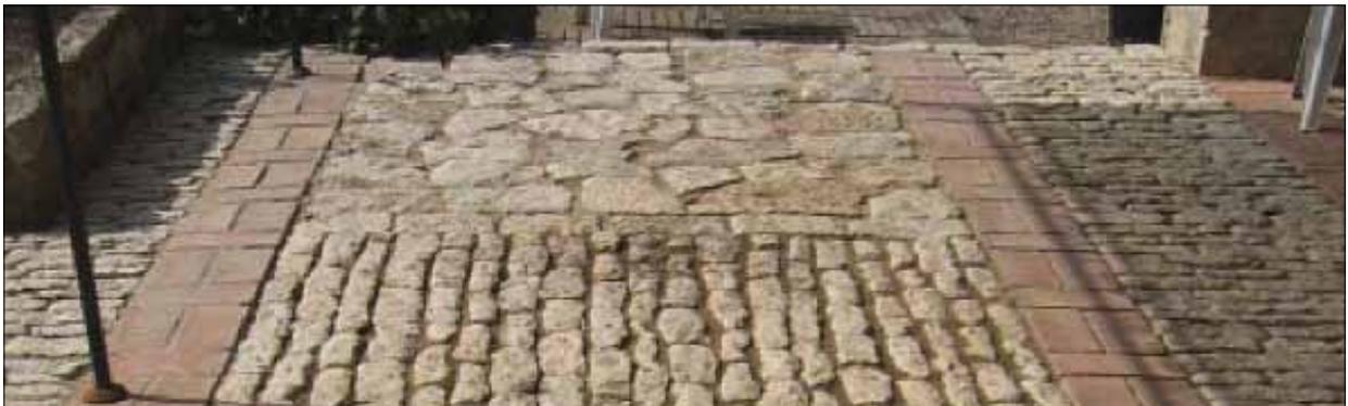
**Wait at least two weeks before putting weight on a pavement with lime. Wet slab daily for 3 days to counter the phenomenon of withdrawal due to premature drying. A mortar made under the sun at a temperature of 30 ° will cause surface cracks as it dries too quickly. A temperature of 20 ° and a shaded exposure are appropriate. Avoid freezing and winter periods. We can tint the topcoat by adding natural pigments (wait for the final drying tests in order to see the color).**
