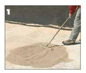
• On own land or on an iron plate (avoid plastic holders), spread 25 kg of quicklime 5 cm thick (Fig.1)
